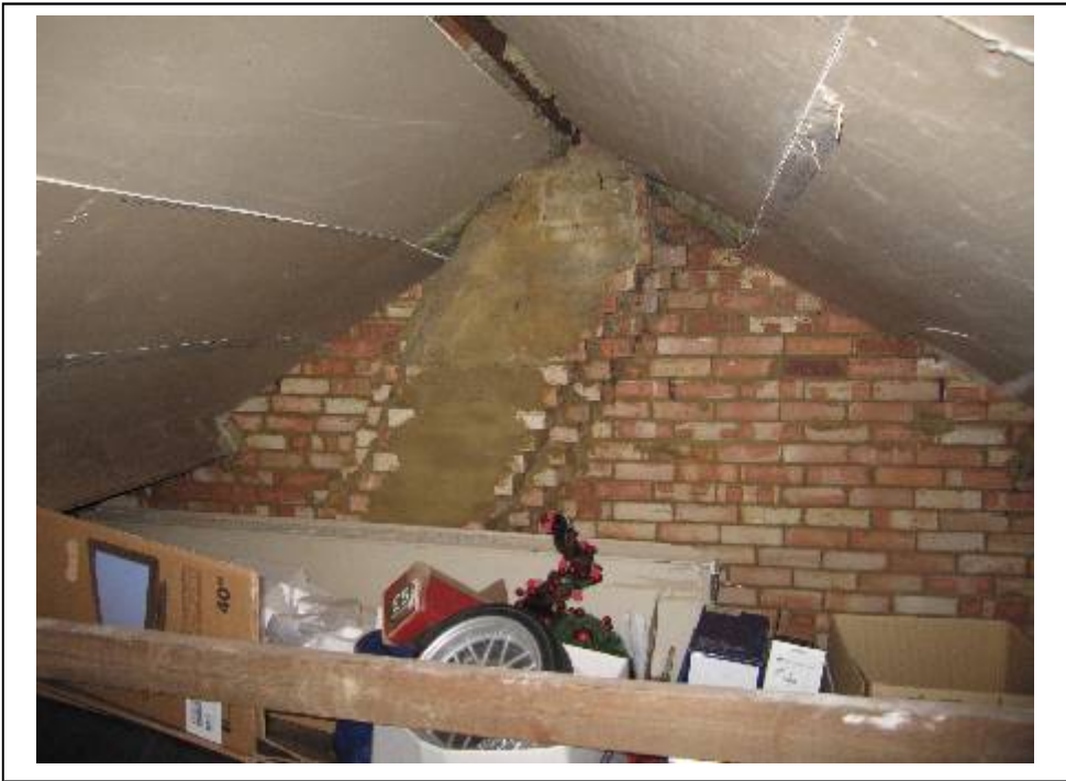
Roof void and party wall
